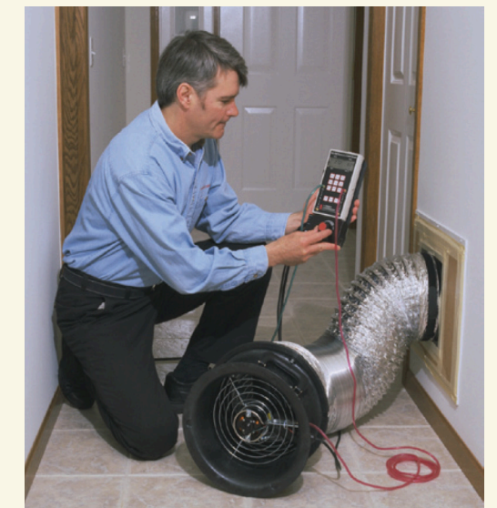
Duct Leakage Test
